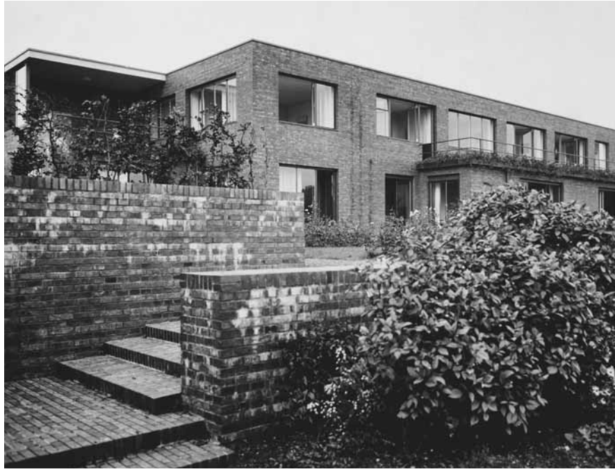
Mies tied the Esters House, right, to the landscape through tiered terraces.
